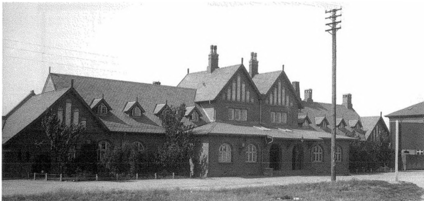
Hernings anden station set fra gadesiden. (Lokalhistorisk arkiv, Herning)
